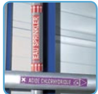
Identify pipe-lines on-site
